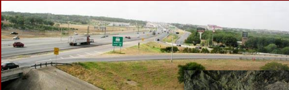
Interchange in the San Antonio suburban (Texas).
